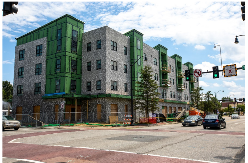
Lift & Rise on Jefferson, Newport News, Virginia. Photo credit: Breedon Construction
