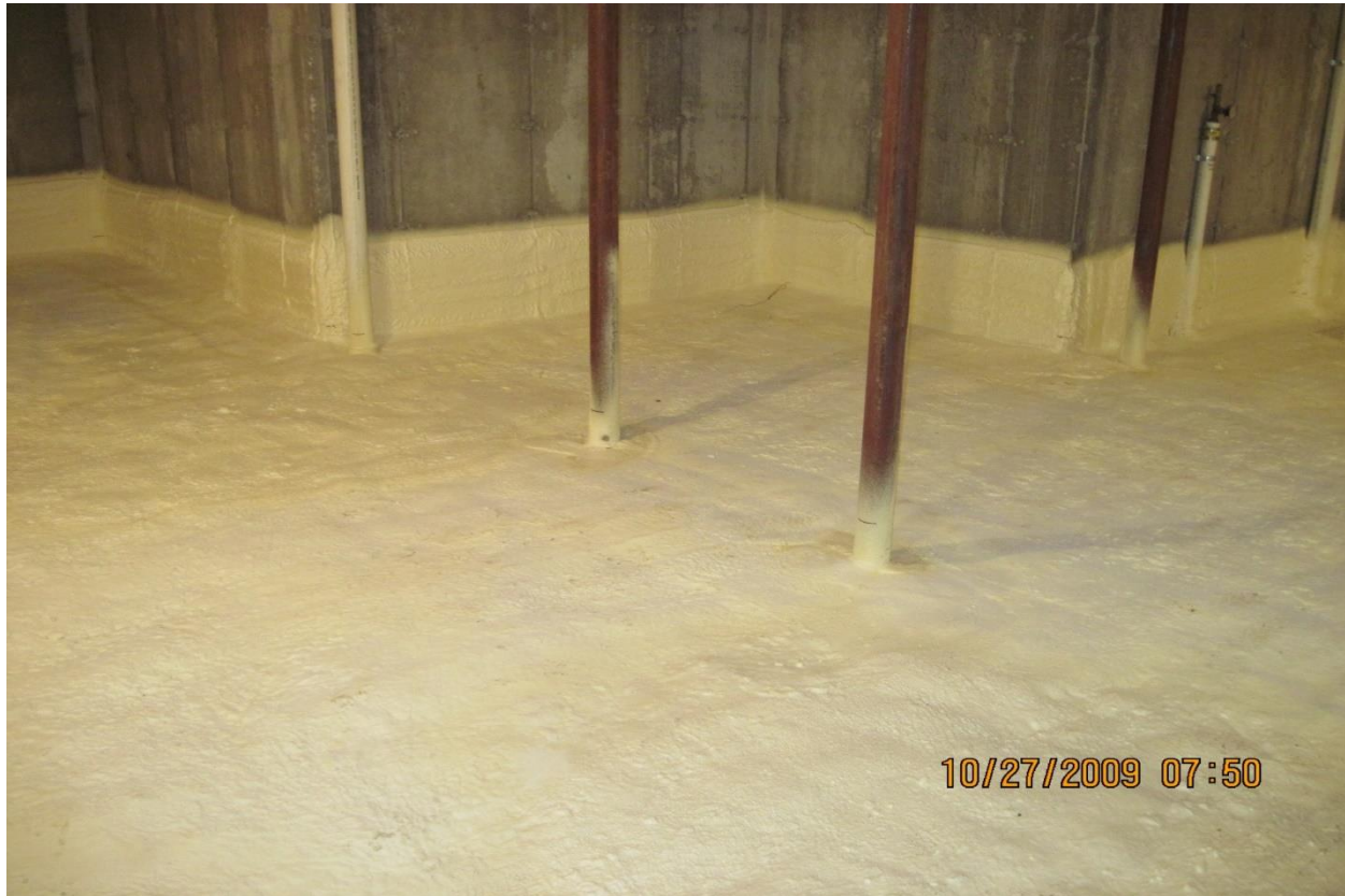
Figure 4 - Sub-Slab Insulation Application (photo)
