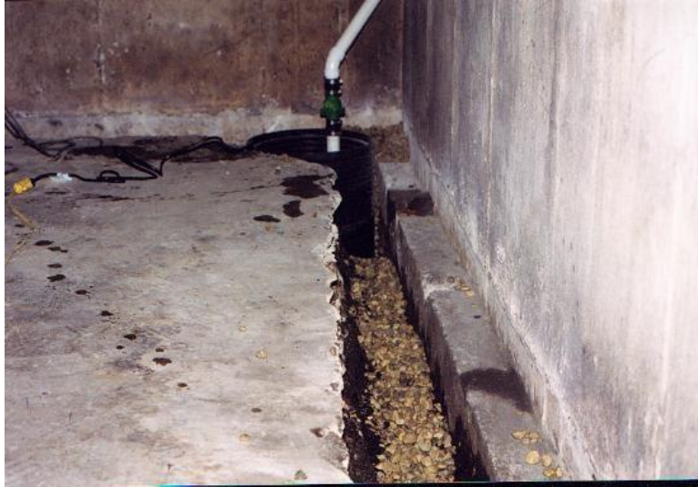
Figure 1 – Interior Foundation Drainage System with Sump Pump
