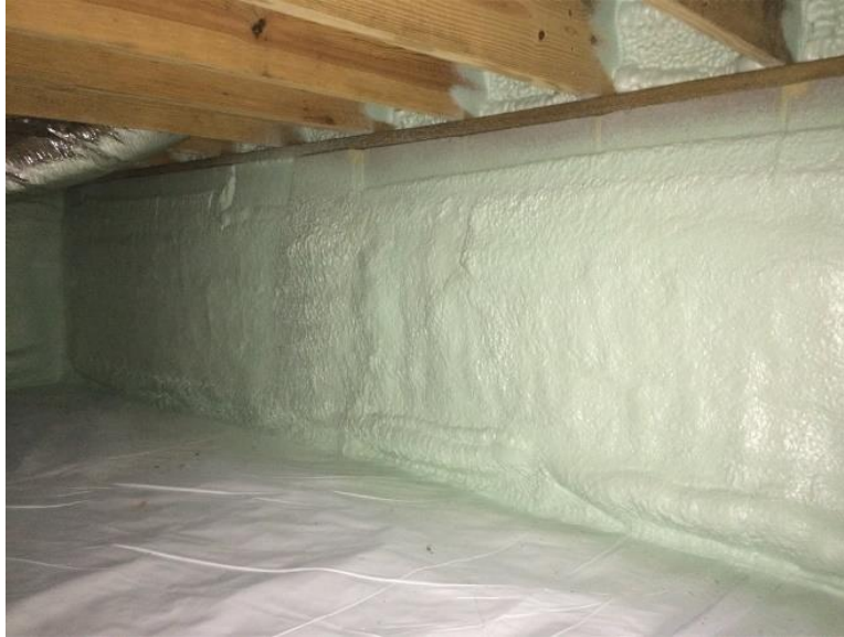
Figure 2 - Example of a Termite Inspection Gap in a Crawlspace Wall
