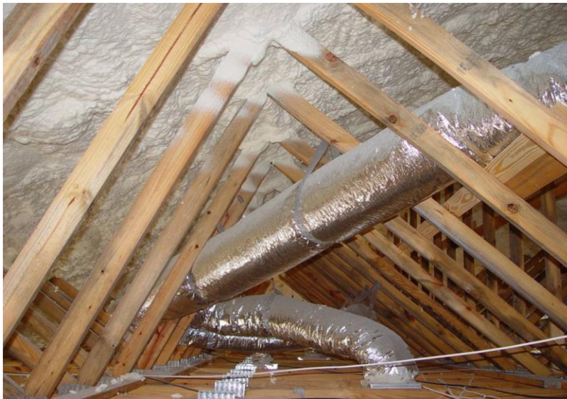
Figure 2 - Actual installation of SPF in an unvented attic. Notice that ductwork is now in conditioned space.
