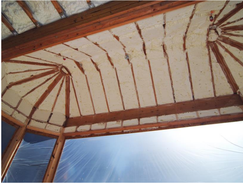
Figure 3 - Actual installation of SPF in a cathedralized ceiling.
