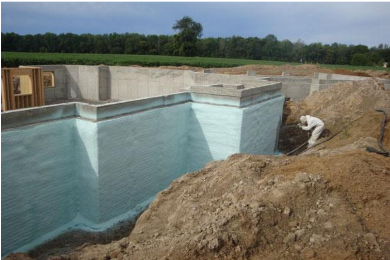
Figure 3 – Exterior below-grade wall installation (photo)
