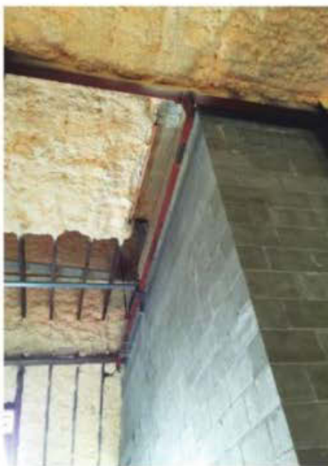
Sprayed polyurethane foam (SPF) offers thermal, air, and moisture control, helping seal the building enclosure with one material to avoid the need to specify numerous additional products to accomplish the same performance.
