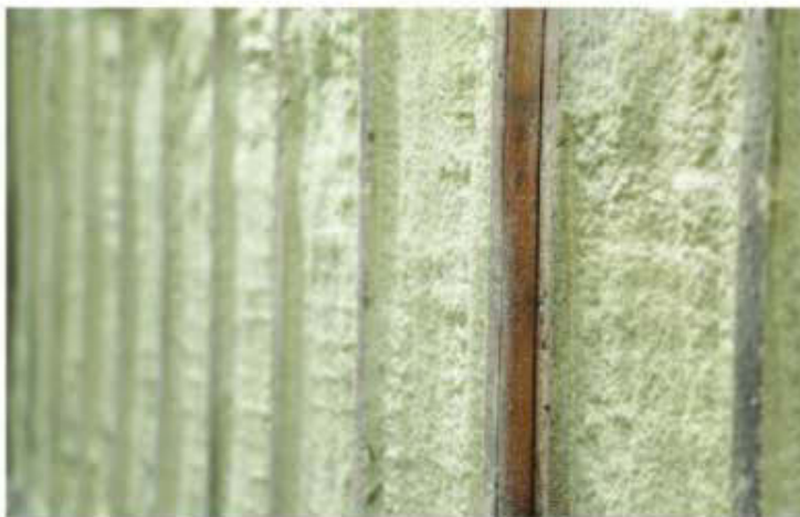
Sprayed polyurethane foam (SPF) offers thermal, air, and moisture control, helping seal the building enclosure with one material to avoid the need to specify numerous additional products to accomplish the same performance.
