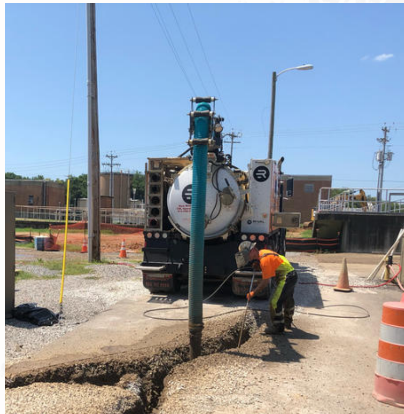
Figure 1: Hydrovac truck used to create a slot trench
