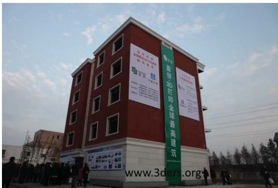
Figure 4 – A 3D printed five-story apartment block (Charron 2015)
