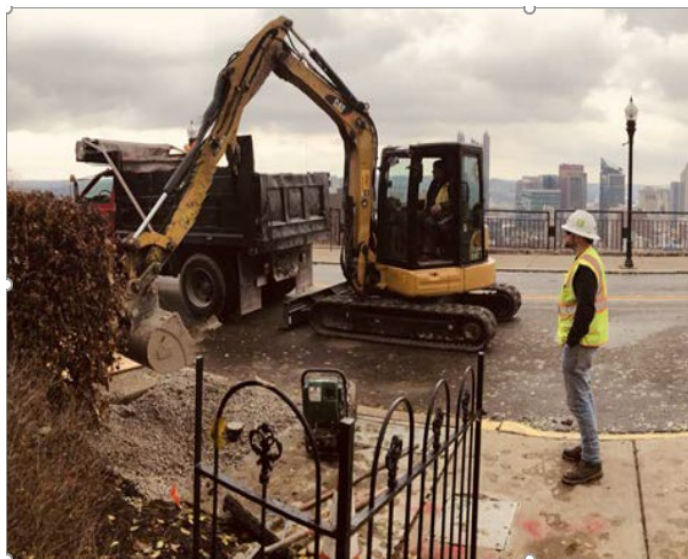
Example of a Mechanical Excavation
