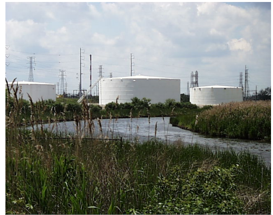
Expanding oil storage capacity may require actions to comply with applicable environmental rules.
