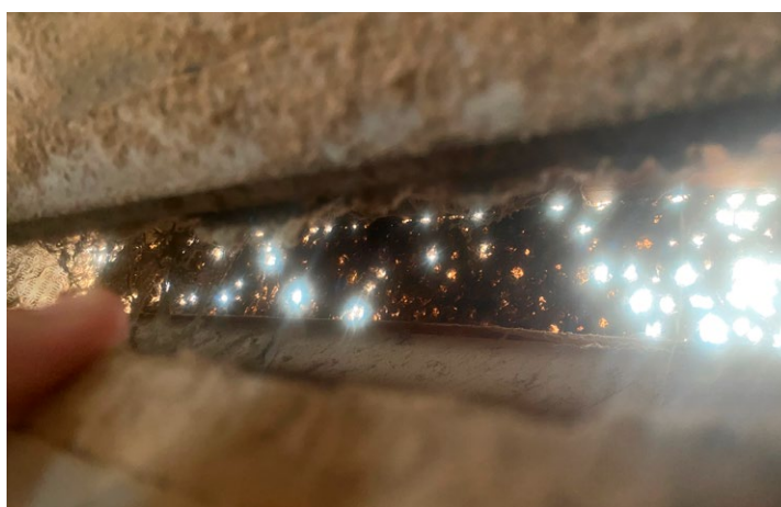
Figure 4: This photo was taken from inside the house looking through the sidewall vent. The bird wire is almost 70% blocked with dust and feathers. It is next to a sidewall exhaust fan. This vent wire is way overdue for a good cleaning.
