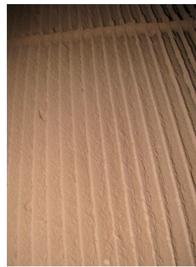
Figures 5 and 6: These photos were taken from a pullet house that was only 5 years old. We are pretty sure the light traps, shutters and fans had never been cleaned. There was about 0.25" of dust on shutters, and about 2.5"-3" of dust settled in the bottom of the light traps and framing. Light traps were totally coated in dust, and about 1-1.5" of dust was in the fan housing. This is a personal foul.
