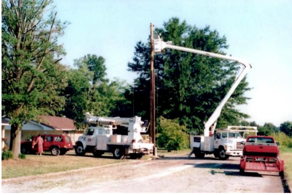
Electric Crew Setting a Pole
