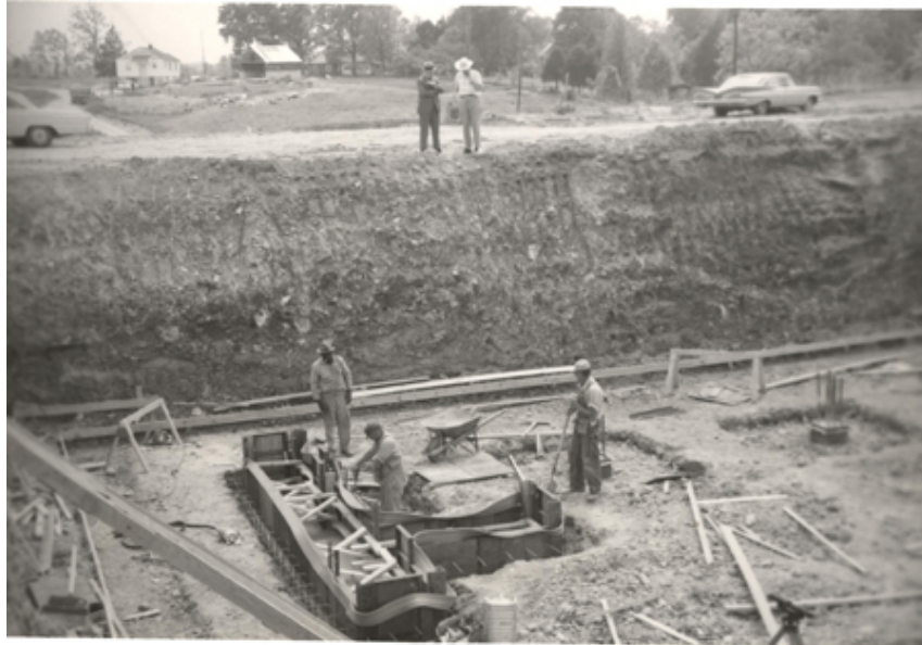
Water Treatment Building Construction 1965
