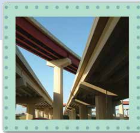
WIDEN EXISTING URBAN FREEWAY $11 million per lane mile
