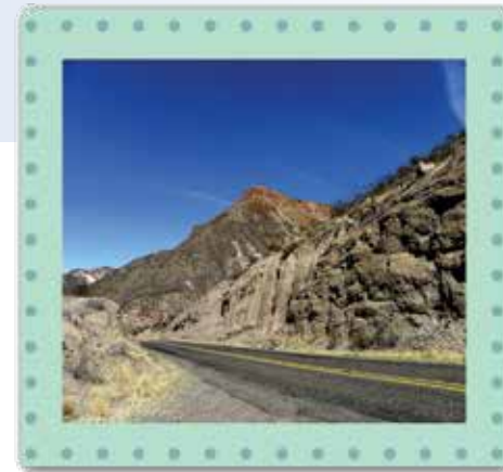
FULL REHABILITATION FM ROAD $1.5 million per lane mile
