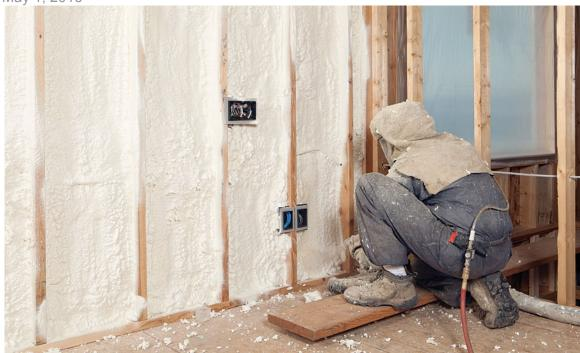
A construction worker is spraying expandable foam insulation between wall studs, near a protected window, at a new home construction project.
