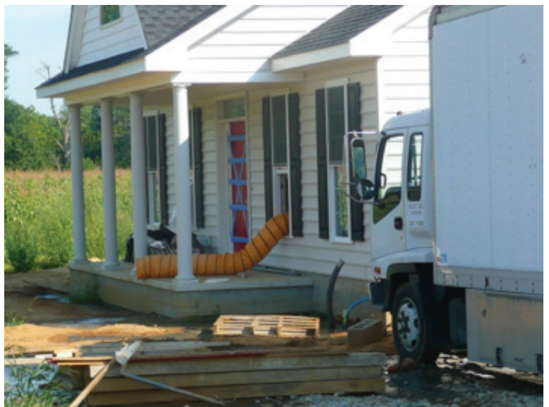
Figure 12: Provide adequate ventilation
