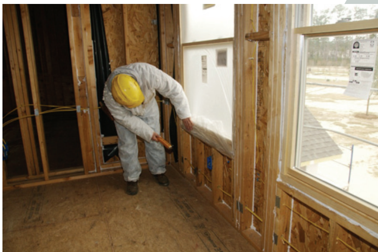
Figure 10: Sealing the windows
