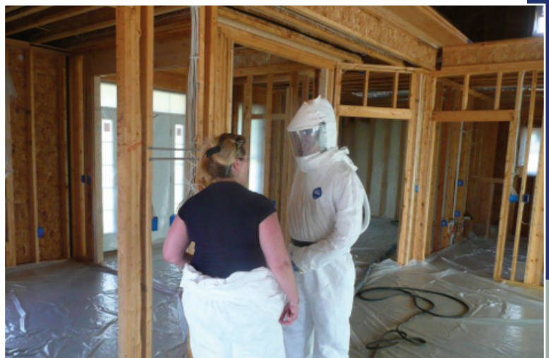
Figure 11: Provide notice to trades and occupants
