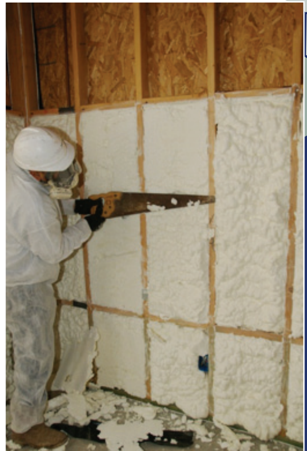
Figure 15: Contractor trimming foam
