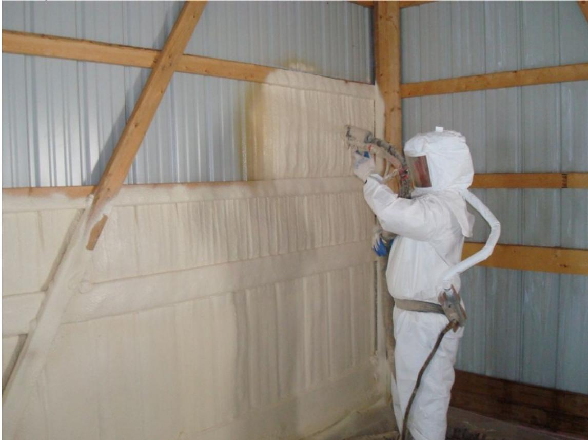
*This photo demonstrates closed-cell SPF insulation applied inside a metal-clad building.*
