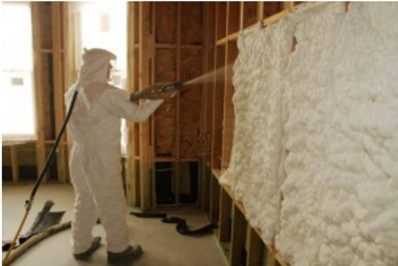
*The installation of sprayfoam insulation in wood framed walls is shown here.*
