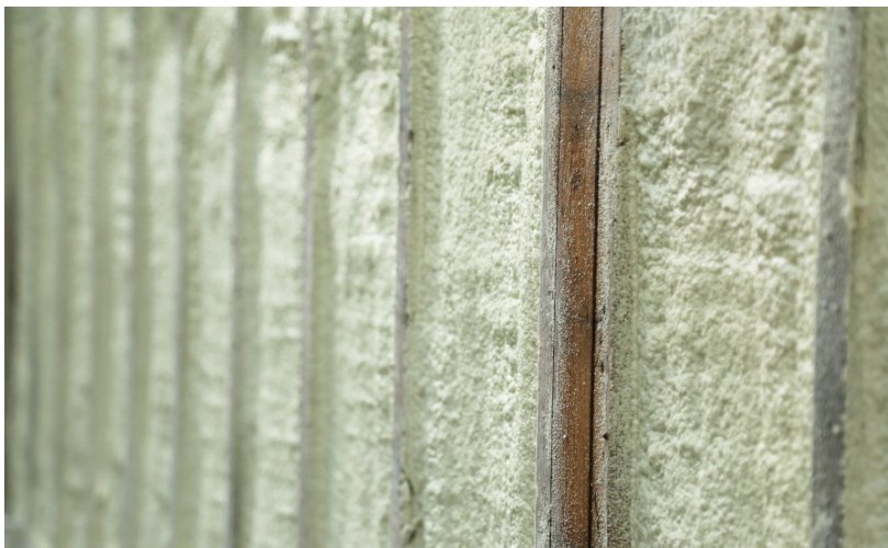
Spray polyurethane foam used as cavity insulation in a wood-framed wall. Photo courtesy of Honeywell.
