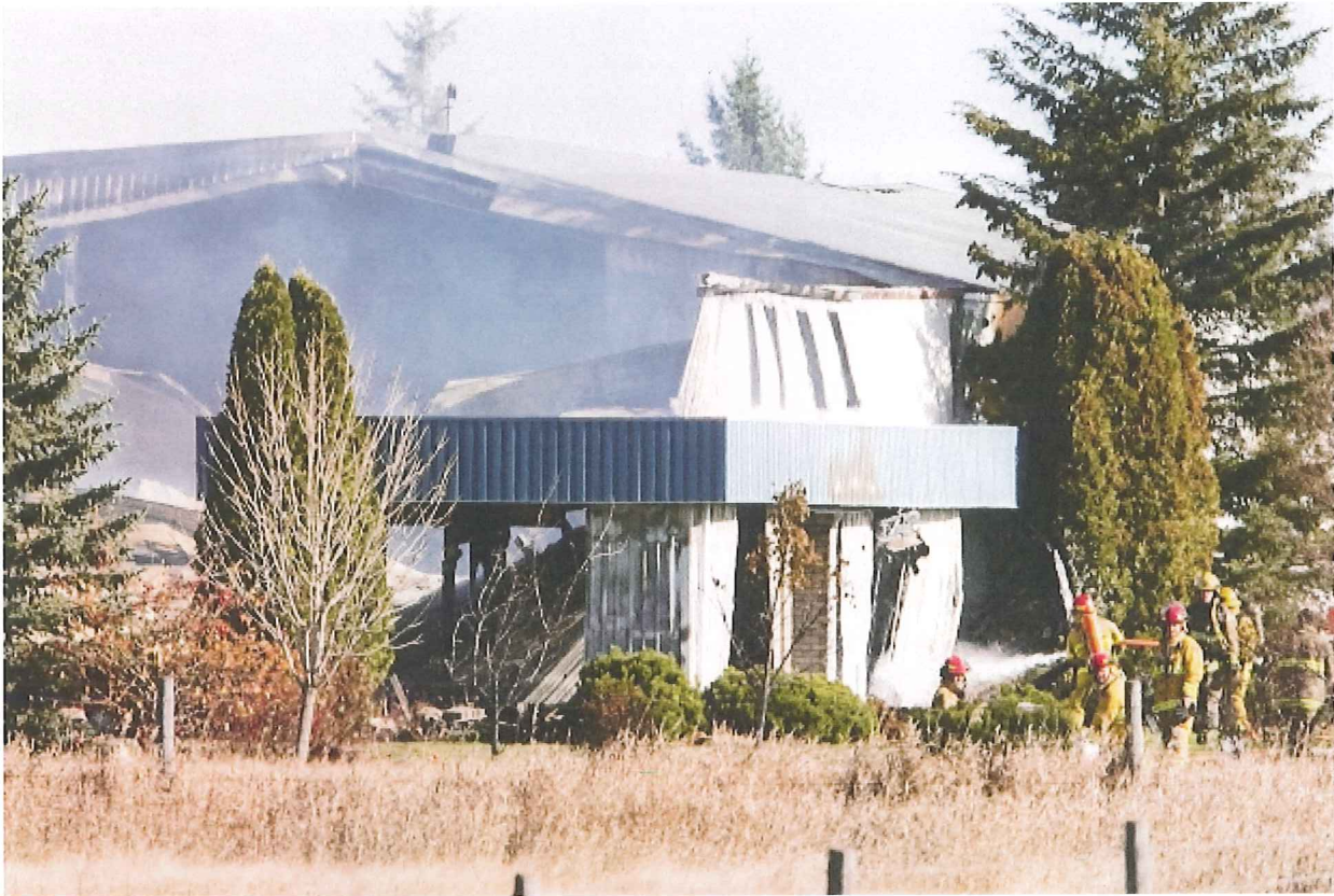
Redekopp Industries west of Saskatoon burned down October 24 2011.
