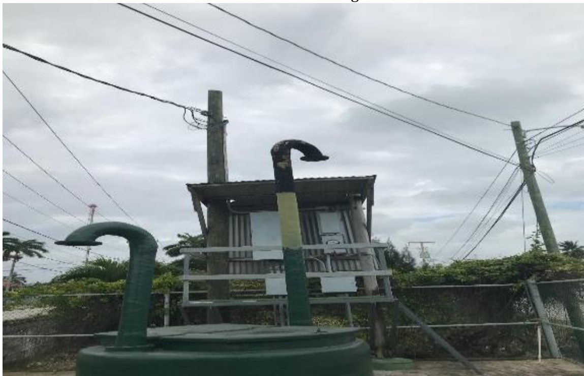
Station N6 – Overhead wires create a hazard for pulling of the pumps.
