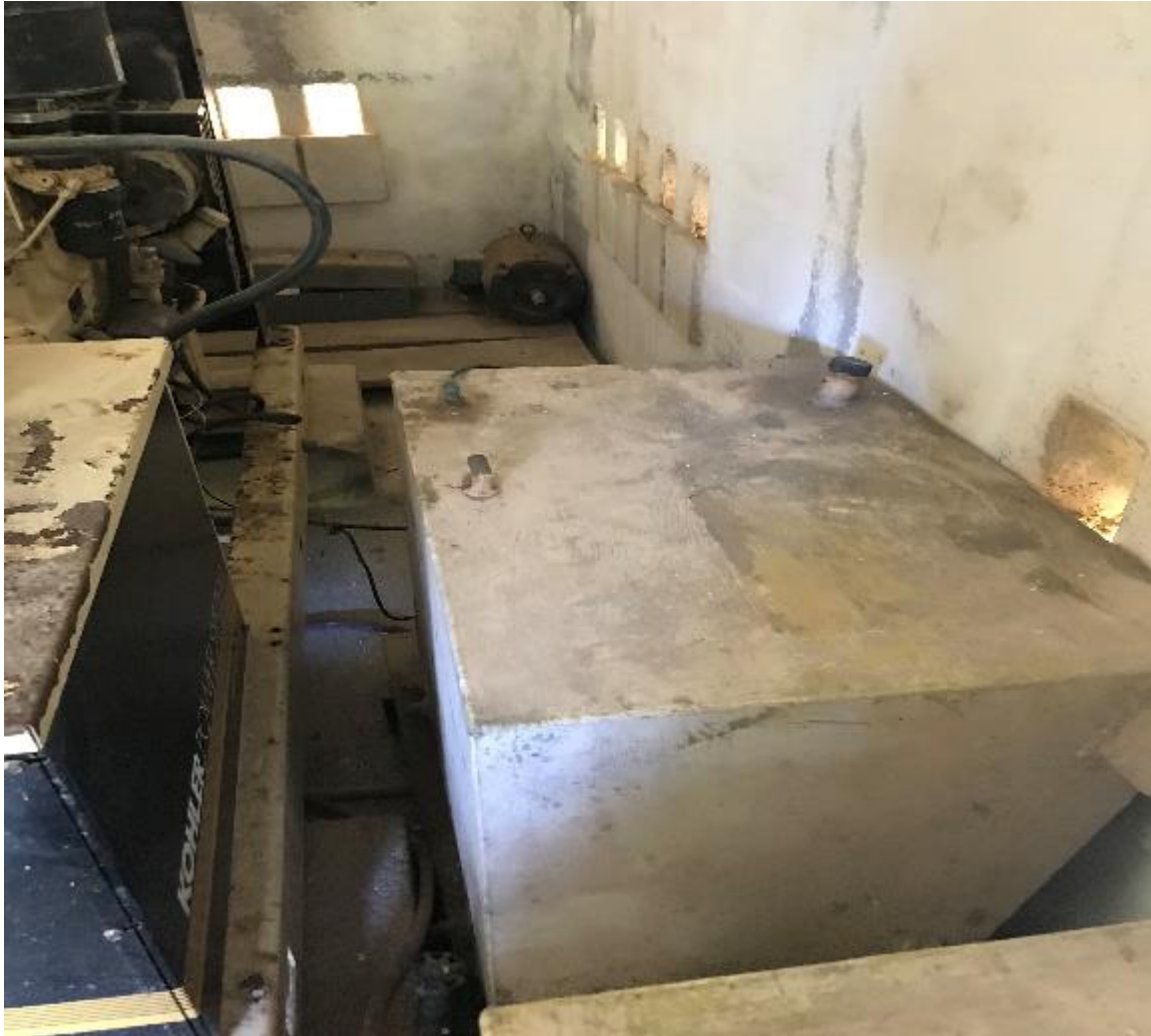
Old single walled tank with limited access and poor containment, evidence of fuel spilled on floor (Placencia)
