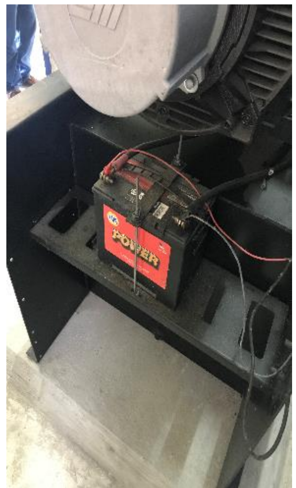
Properly sized batteries but requires protection Small single battery
