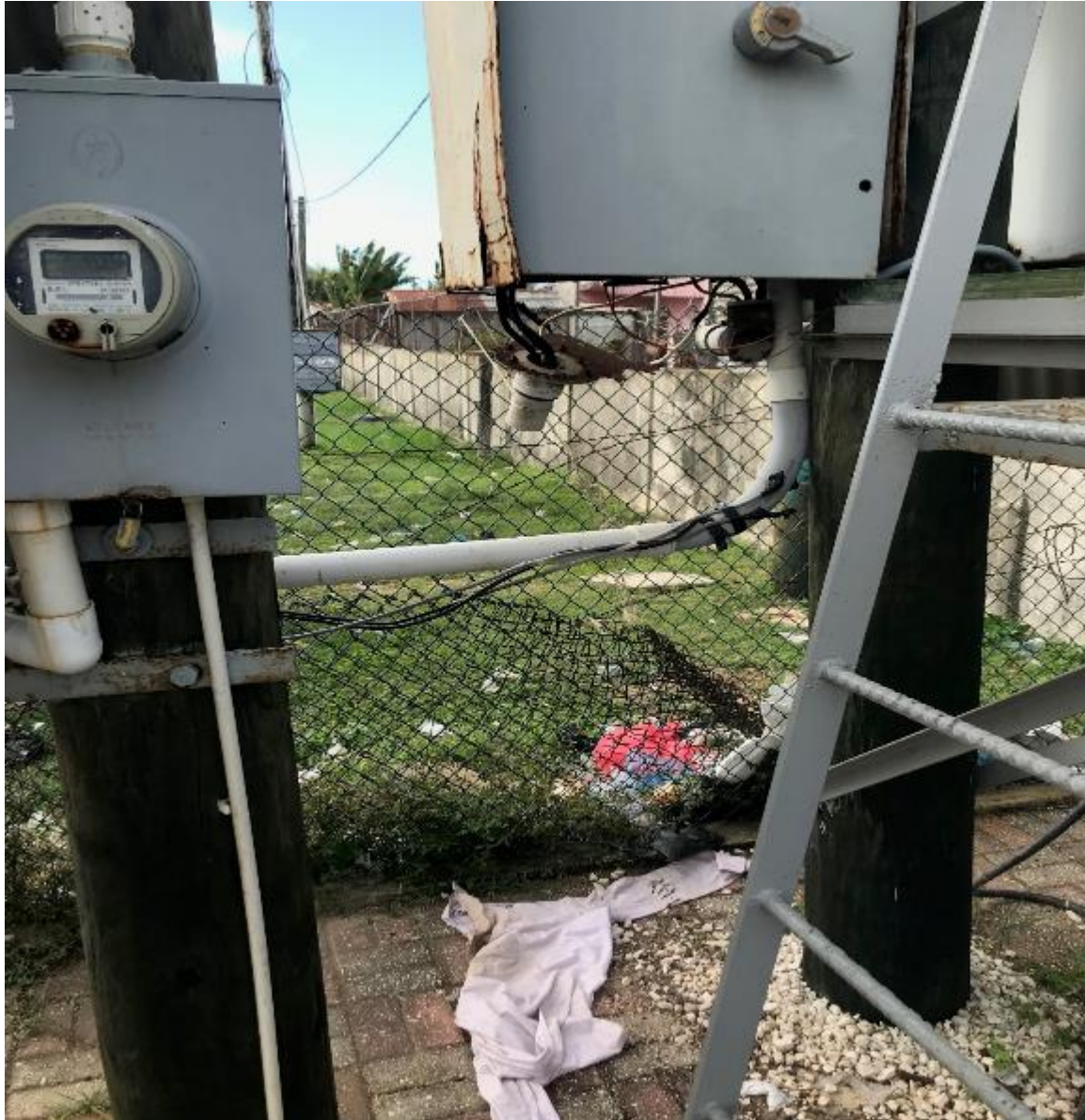
Exposed electrical for generator connection at N3.
