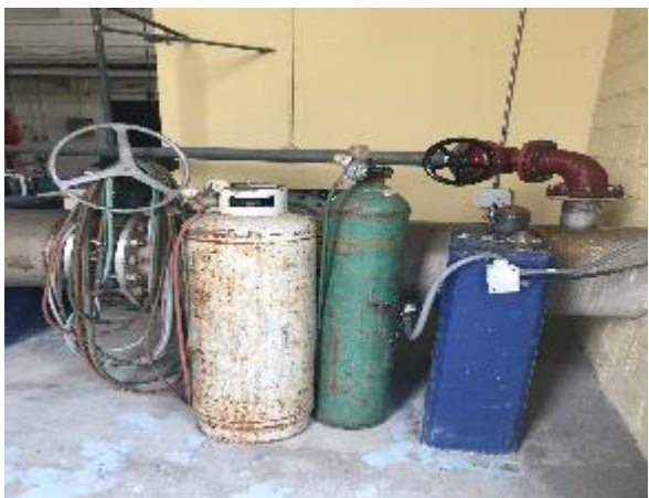
Chain compressed cylinders in place - Do not block electrical panels or controls
