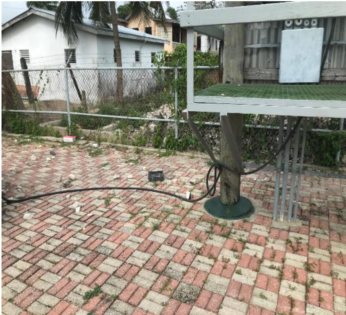
Exposed pump power cable.
