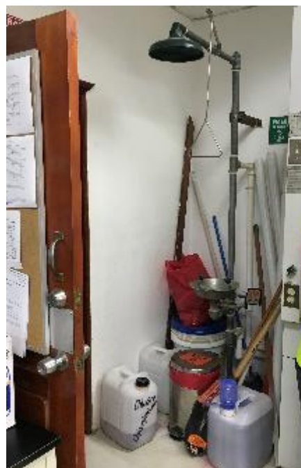
eyewash blocked in lab area
