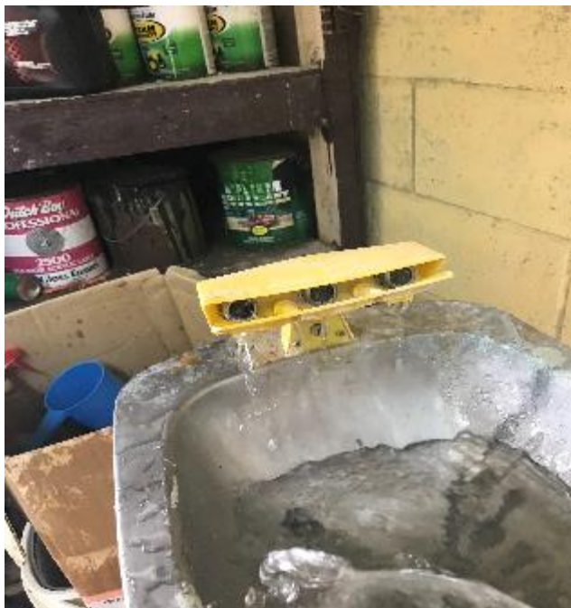
Nonfunctioning eyewash doublerun
