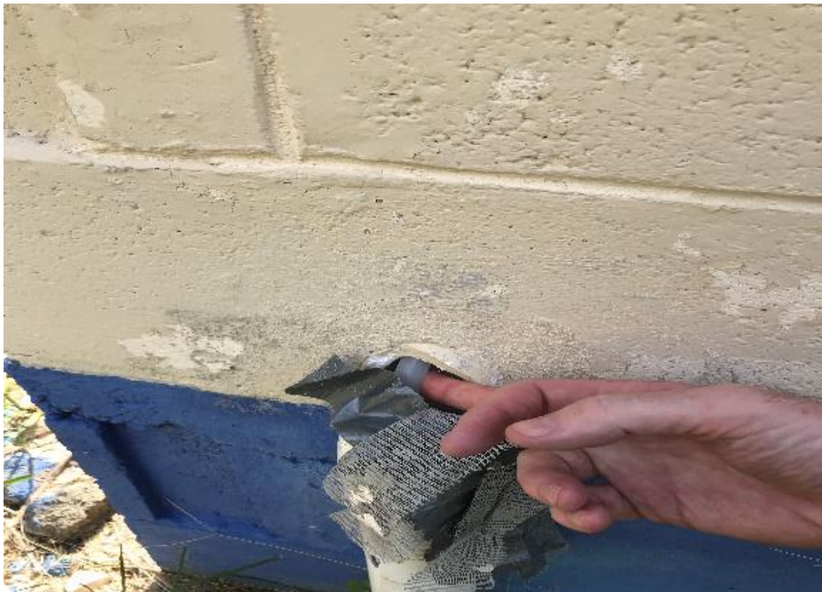
Chlorine injection line exposed at back of building
