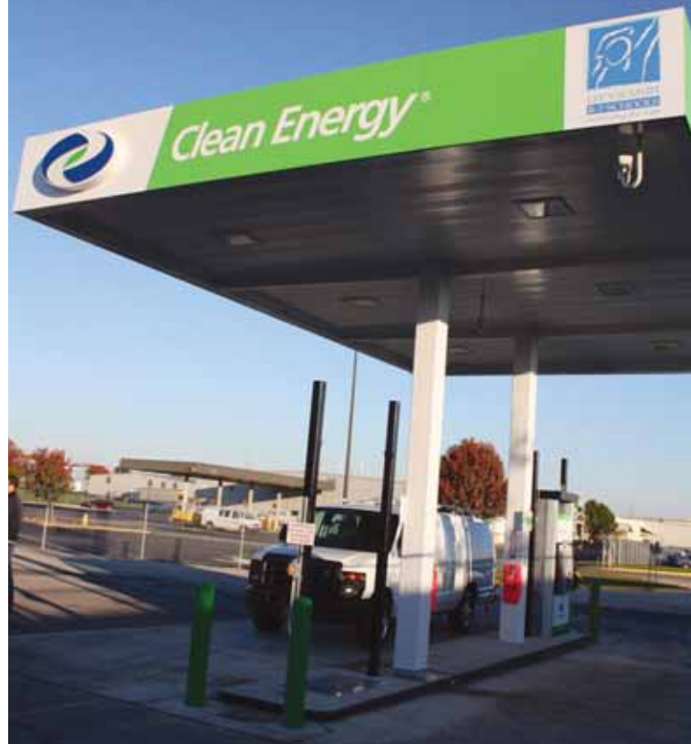
Public CNG fueling stations keep the community running.
