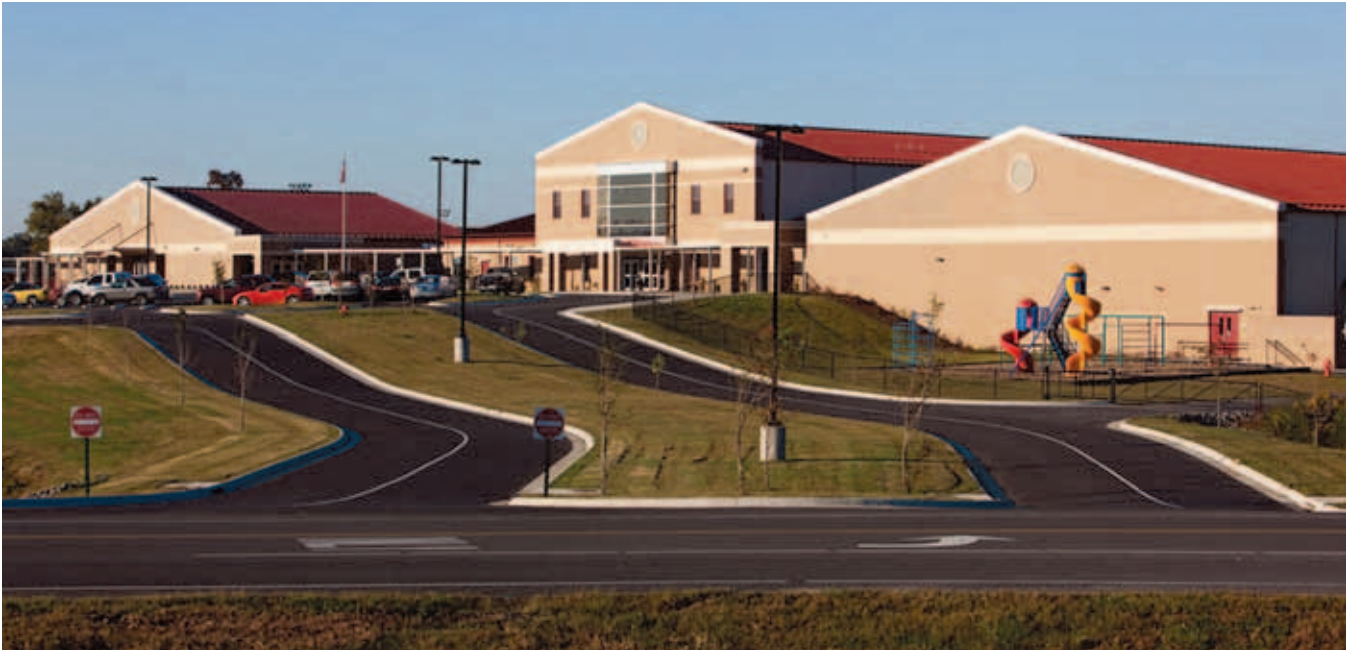
Lake Hamilton Intermediate School in Hot Springs, Arkansas, takes advantage of the benefits of metal roofing.
