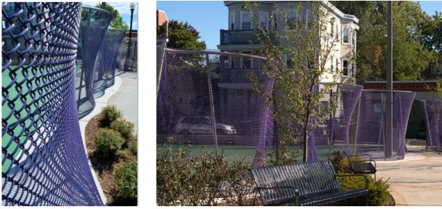
The project consists of a sculptural fence made of chain link fabricated in a serpentine sharp with sinuous curves. In this fence, the top and bottom rails are serpentine, and the pother posts are set purposely at angles to create a sense of rhythm and energy. The chain link fabric is stretched around the structure to create billowing curves.
