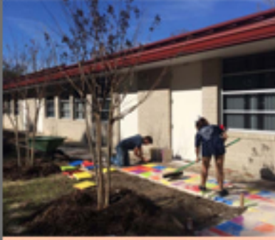
SCASLA members almost finished at Irby, polishing up the pavers
